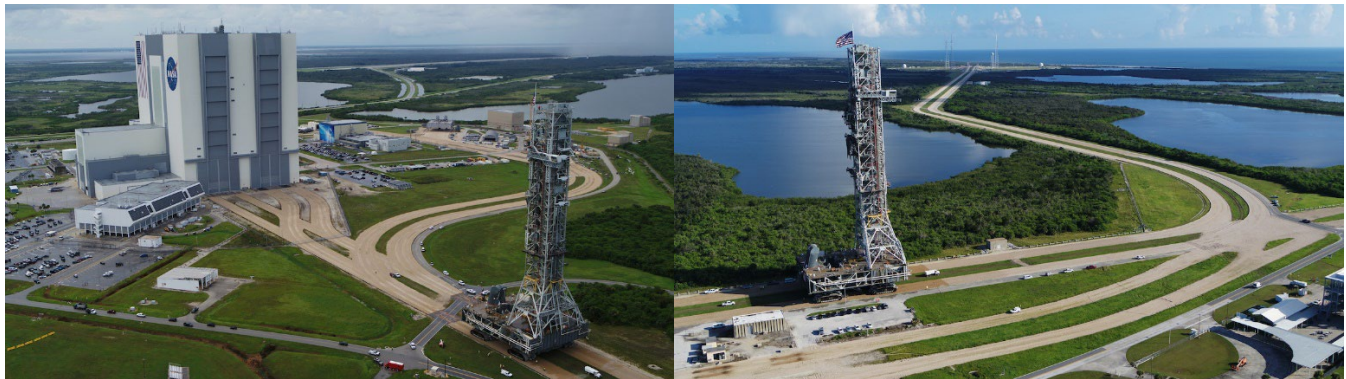
Figure 7. ISVV-005 Rollout September 2018.
