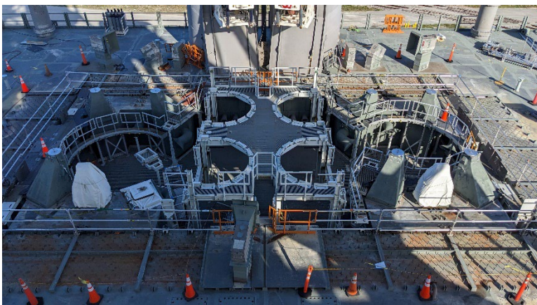
Fig 3. Zero Deck Showing 7 VSPs Post Artemis I Launch
