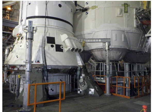
Fig 2. Mobile Launcher 1 Zero Deck Showing VSPs
