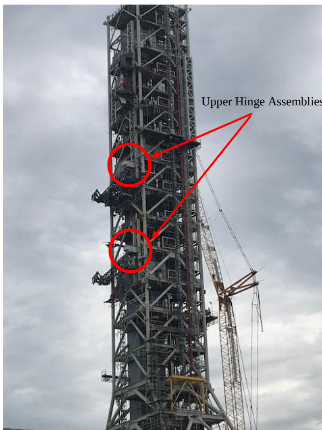
Figure 1. Two upper hinges mounted on ML.
